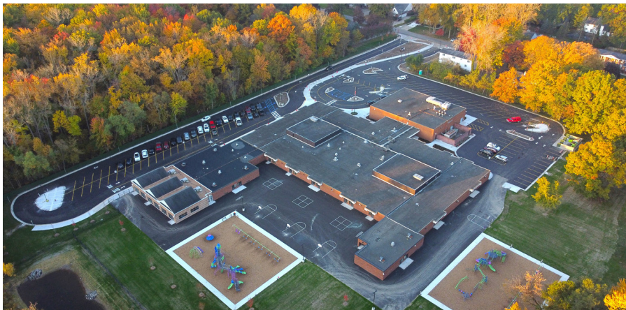
The Crissman Elementary School parking lot was redesigned to improve safety by separating the bus loop from the parent/guardian drop off area. Improvements at Crissman also included the installation of new playgrounds.
